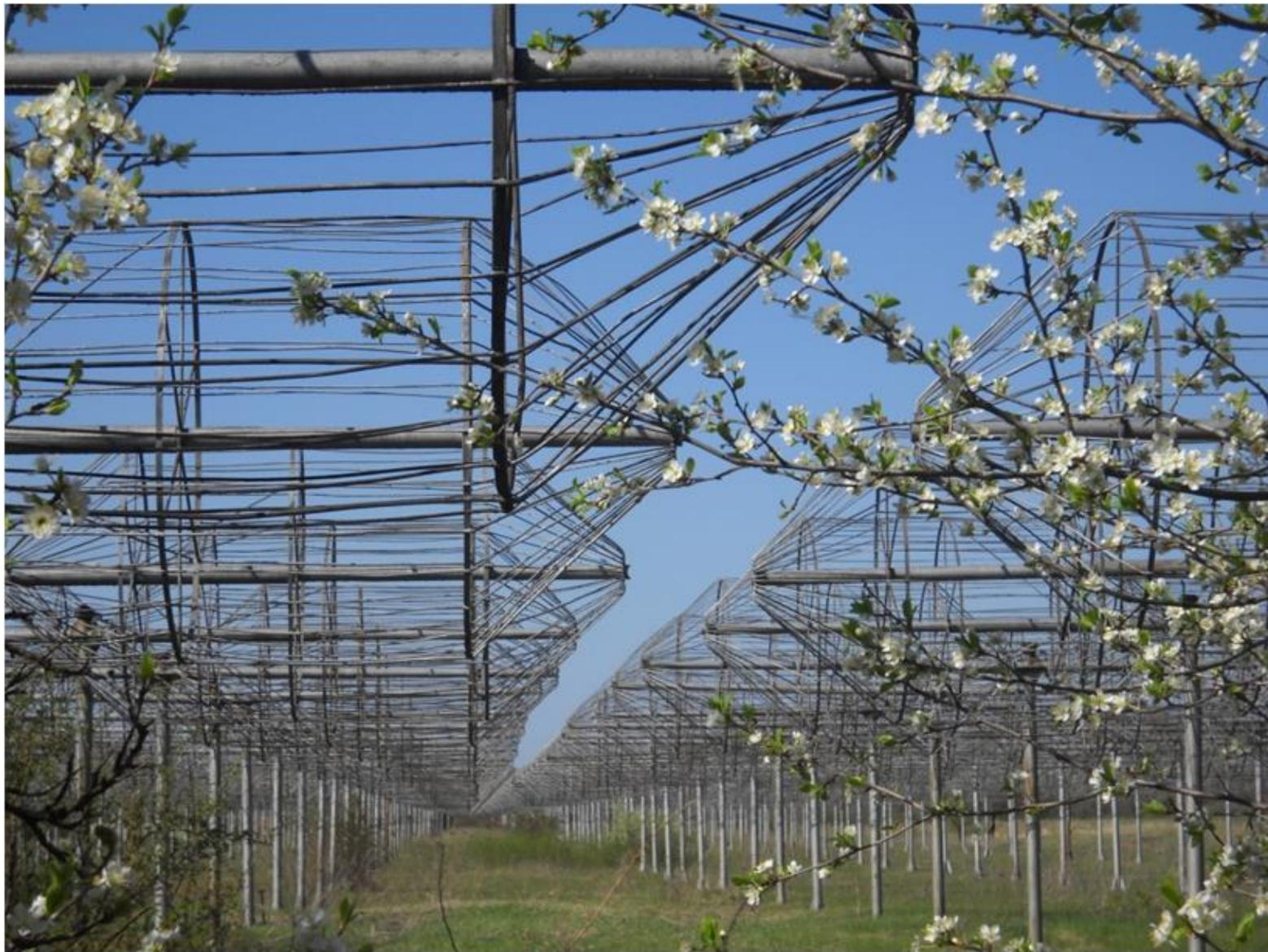
**The world's largest UTR-2 radio telescope (N-S arm, 1.9 km x 60 m)
