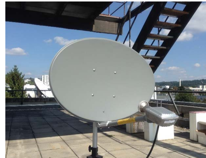
VSAT with 74 cm dish size: the typical ground terminal antenna
